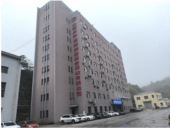
驱动机房南侧联合建筑
